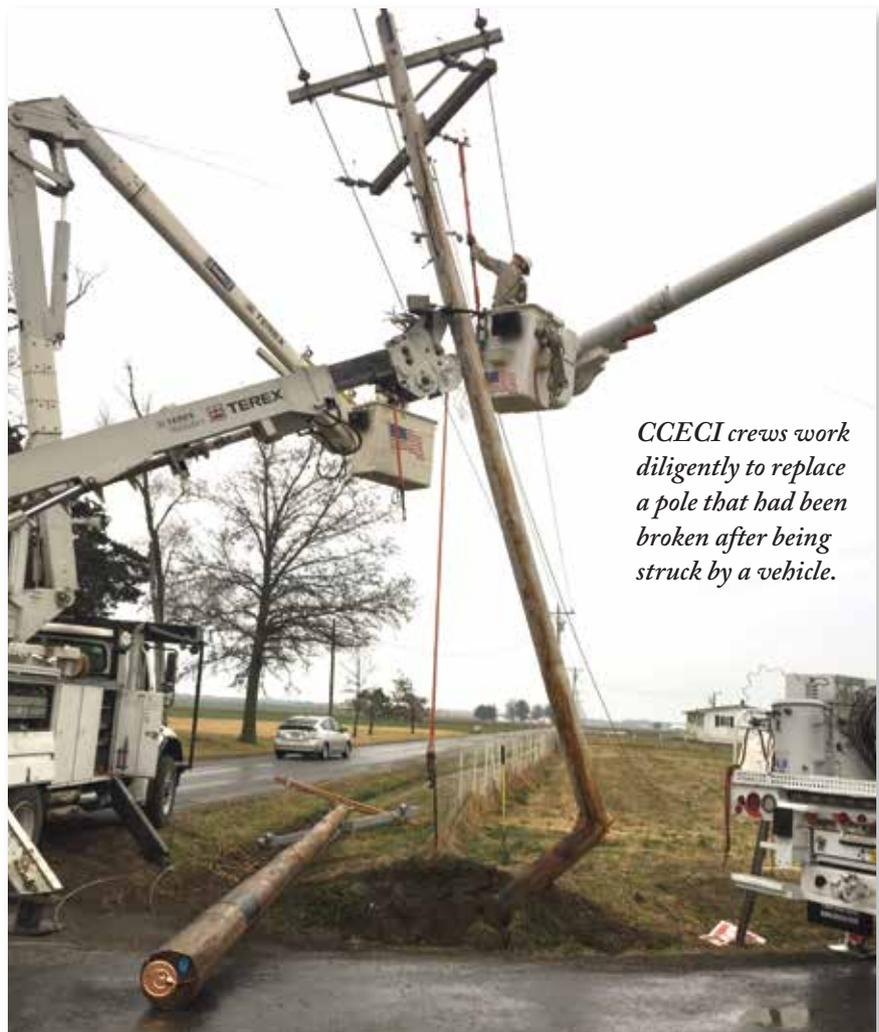
*CCECI crews work diligently to replace a pole that had been broken after being struck by a vehicle.*
