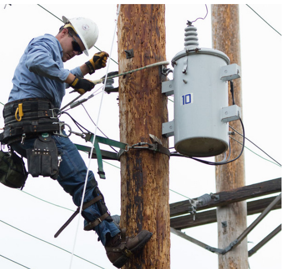
Apprentice Lineman Justin Hubert is doing his part in the H-Structure Obstacle Course.
