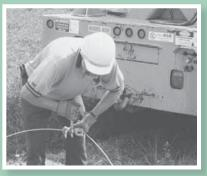
Lineman Allan Deiters tightens a piece of hardware called a "deadend shoe." The dead-end shoe is used to hold overhead wire at the beginning or end of a line. The only thing that holds the wire up after the shoe is hung from the pole, is the clamp that Al is tightening, so he bears down on it to ensure the wire won't slip out.
