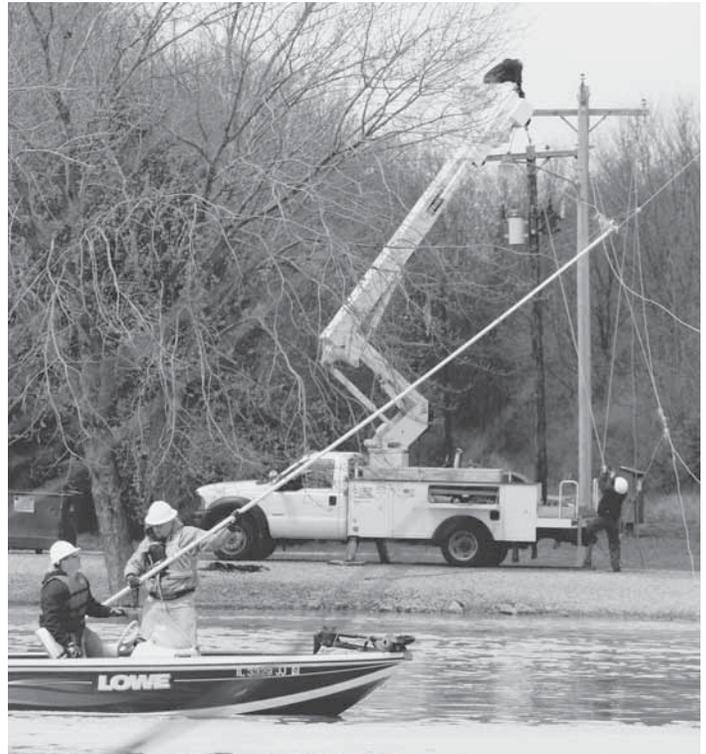
Journeyman Lineman Brian Taylor and Apprentice Lineman Mike Faust braved rushing currents, frigid water, and cold winds to board a boat below the spillway at Carlyle Lake and repair a damaged three phase line that mysteriously became tangled together on April 13th. The first and longest step in the repairs was to remove years of tangled fishing lines from the wires so they could be separated and re-hung. Pictured are Taylor and Faust fighting the currents and the knots of fishing line.
