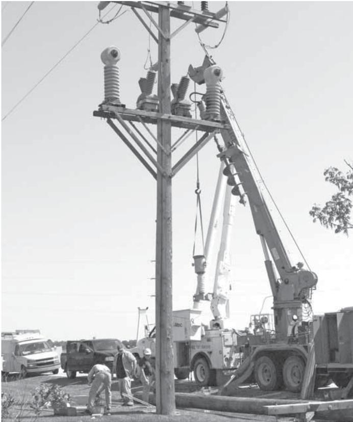
On May 21, CCEC Linemen assisted Big D Electric in performing maintenance to a transmission line that feeds the two substations that provide power to the southeast corner of our service area. Big D Electric changed out a 65-foot pole near the intersection of Highline Road and Shattuc Rd, while CCEC crews changed out some defective hardware in CCEC's Shattuc #1 Substation.
