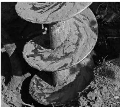
*The hole from the old pole is augered out to make space for the new, larger pole. The auger is carefully positioned as not to damage the existing underground cables that will need to be attached to the new pole.*
