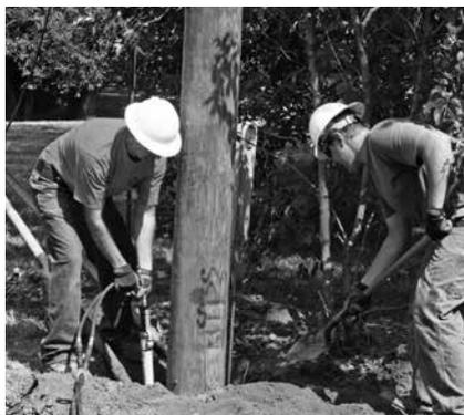
*While the linemen in the bucket pulls the energized conductors out of the way, the new pole is swung into place, guided into the hole, and the backfill is tamped to keep the pole straight.*
