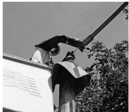
*The energized lines are guided onto the new insulators and tied down.*
