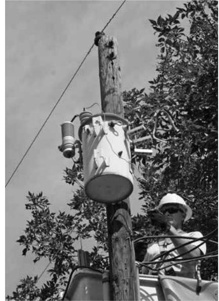
*The old equipment and wires are removed from the rotten pole. The 7200 Volt primary line is kept energized while it is removed to minimize the number of customers that will be out of power.*
