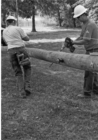
*Holes are drilled in the new pole to allow for bolts and other equipment to be installed on the pole.*
