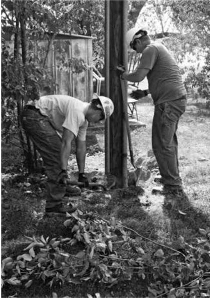
*The underground wires that run down the side of the poles are exposed by hand digging, also allowing the existing riser pipes that encase underground wires to be maneuvered to allow for the new pole to be set in place.*
