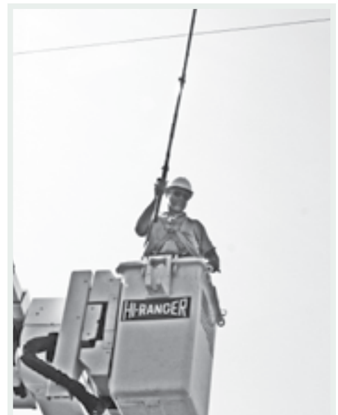
Leadman Lineman Allan Deiters installs fault indicators on a line near New Baden. The indicators will assist the linemen in finding faulty equipment that has been making the power flicker in this area.
