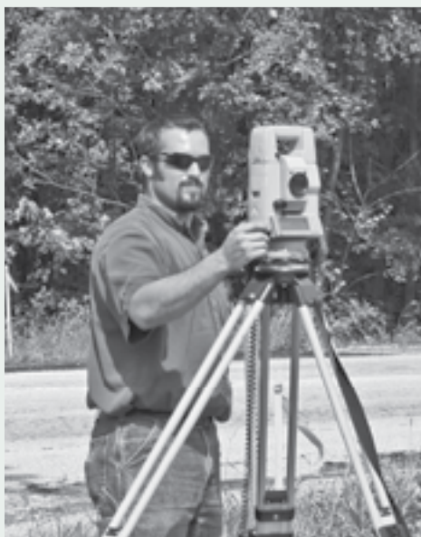
Engineer Bob Kroeger and Operations Assistant Ahren Langhauser stake out new pole locations near the intersection of State Route 161 and Shattuc Road. The engineering department is always updating their work plans to keep up with constant maintenance that is needed on the electric distribution system.
