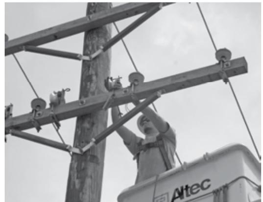
▲ *Here a Big D Electric crew member is installing stringing pulleys to the newly constructed cross arm.*
