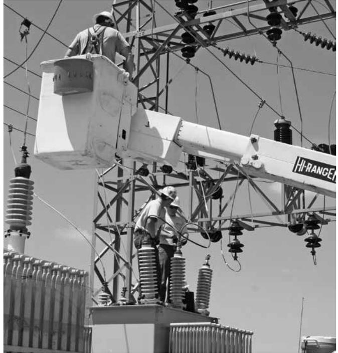
*These pictures show CCECI linemen replacing 3 old 833 KVA transformers, with 3 refurbished 1250 KVA transformers at our Bartelso Substation. Increasing the transformer capacity at the Bartelso Substation should allow for growth in the many years to come.*
