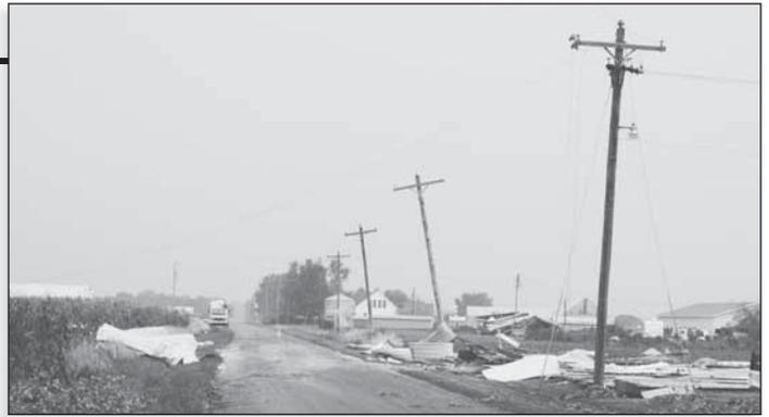
A three-phase line west of Germantown was torn down from an old chicken barn being blown into it. As you can see, high winds and flying debris leaned the pole over and ripped the wire from the top of the pole.
