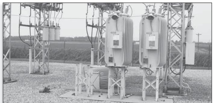
Two of the three voltage regulators in Albers Substation survived the intense winds produced by the storm. The A Phase regulator was blown off of its stand by the high winds. The regulators weigh around 2200 pounds each and contain 115 gallons of mineral oil to keep them cool during operation. Notice the corn that surrounds the substation was almost flattened by the wind.
